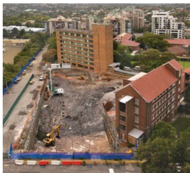
Excavation is underway – picture taken 9 March 2007
